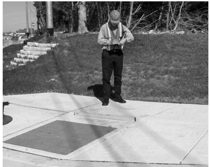
**Using “smart level” to measure cross slope of ramp**
