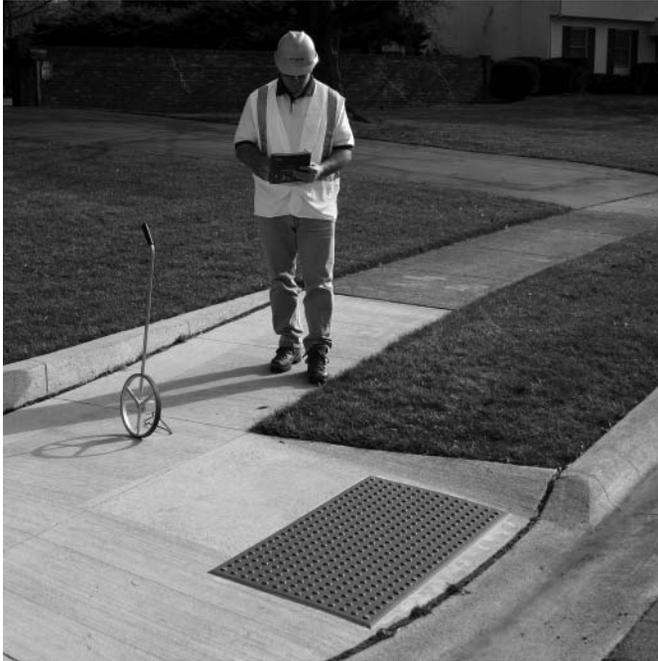
**Inspecting truncated dome installation for detectable warning component of ramp**
