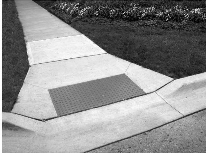
**The above photo shows a compliant curb ramp. Components include detectable warning, sloping ramp surface, side flares and landing area at top of ramp for maneuverability.**
